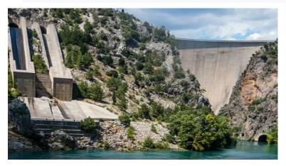
**Oymapınar Dam:** It is a dam built on the Manavgat River in Antalya between 1977-1984 for the purpose of generating electricity. Oymapınar Dam has an imposing and impressive appearance with its height of 185 meters.
